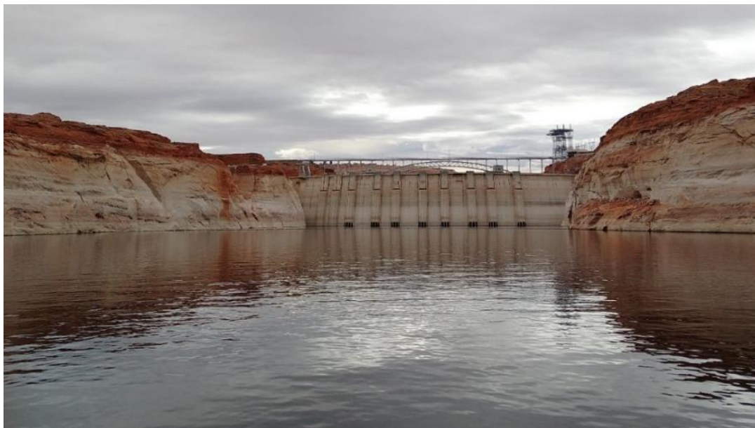
Fig. 4. Glen Canyon Dam. Photo by the author.
